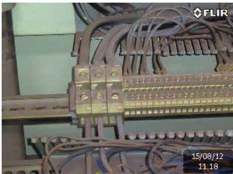
A conspicuous cable or terminal can be detected here. The system operator should inspect the cause.
